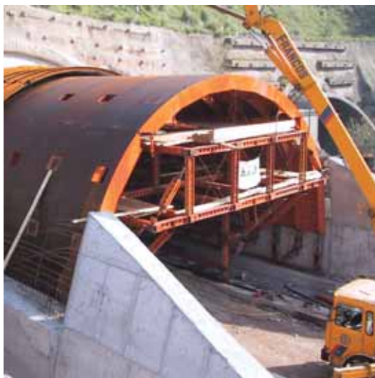
Client: ELSAN - SACYR Project: Tunel Sierrapando, Spain. Rail mounted 6.5m radius steel tunnel form, 12m long, supported off a Super Slim Soldier assembly.
