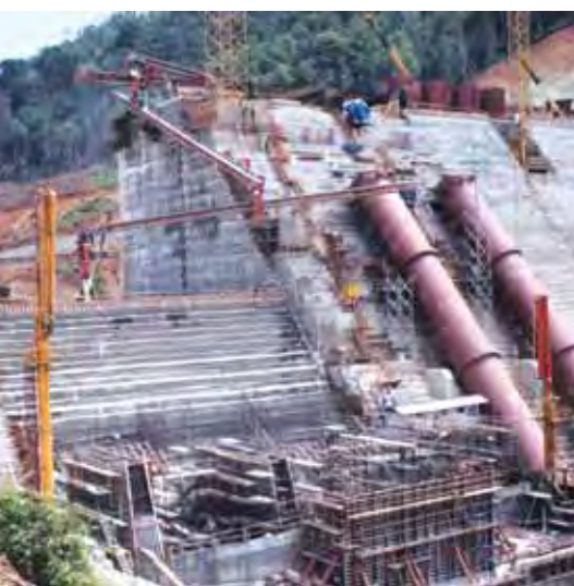
Project: Balambano Dam Project, Soroako, Indonesia, for Astaldi Thiess JV.
