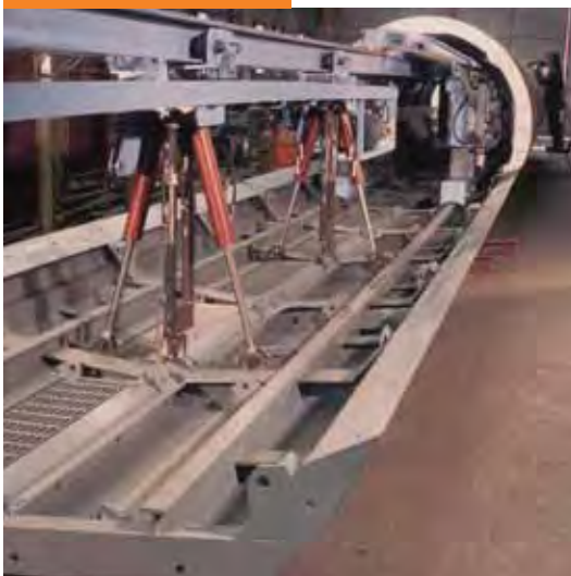
Client: Elanteam Universale Bau Project: Diversion Tunnel, Sungai River, Kelinchi Dam, Malaysia. 9.6m tunnel form made up of Flexform panels on custom made circular steel ribs, light enough to be erected by hand, due to no crane access on site.
