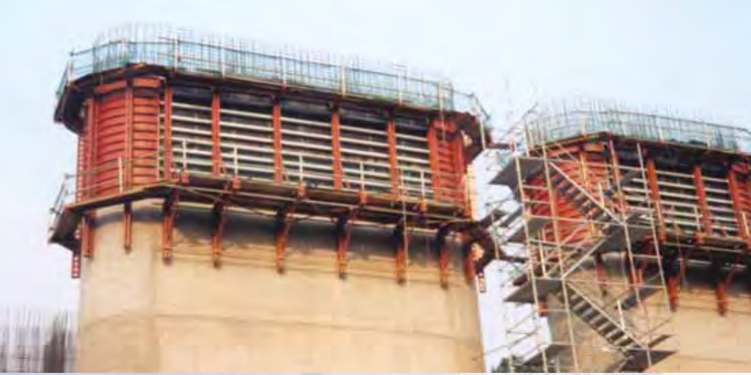
Special bull nose pier jump forms for multiple lift pier construction.
