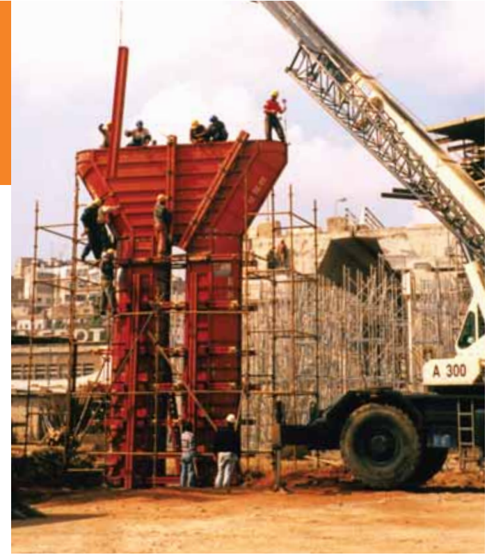
Steel hammer head side and soffit Special formwork supported from adjustable jacks anchored to the pier.
