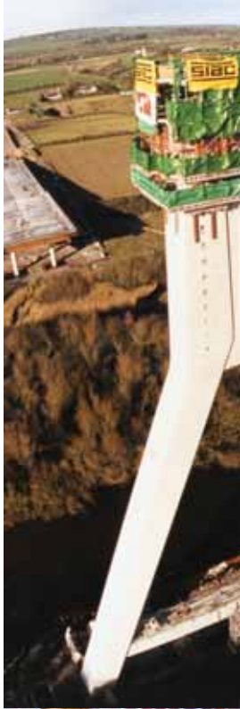
Client: SIAC / Cleveland Bridge Joint Venture
