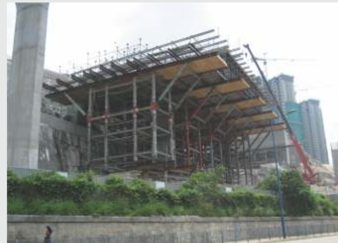
Choi Wan Road / Jordan Valley Bridge - Hong Kong
